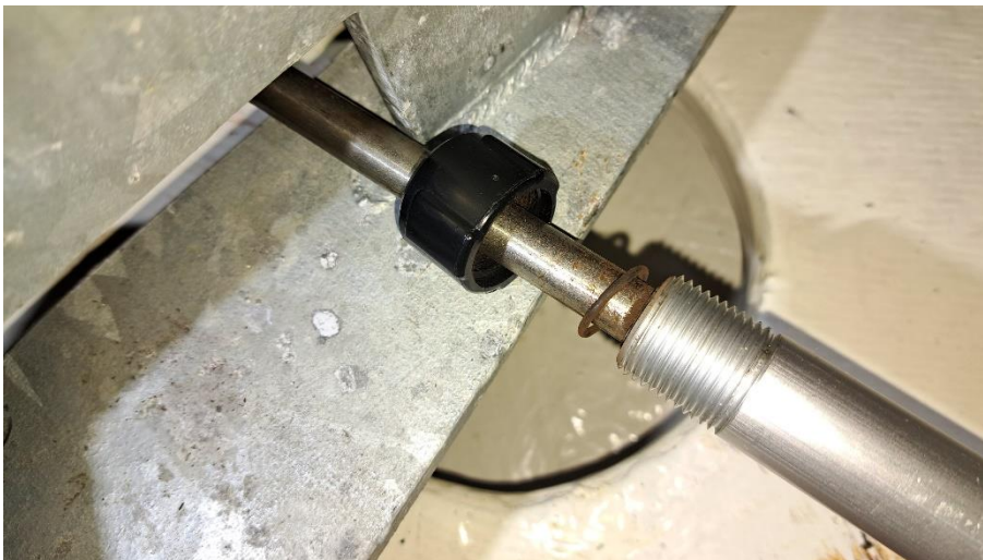
Pic 3: Black plastic cap and the hidden o-ring at the end of one of the threaded tubes
